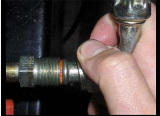
Align fittings and ensure seal is seated correctly.
